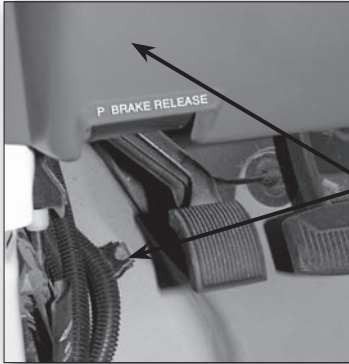
E-450 Charge System Fuse, located behind panel & Rear Ignition Power Fuse (shown with kick panel removed)
