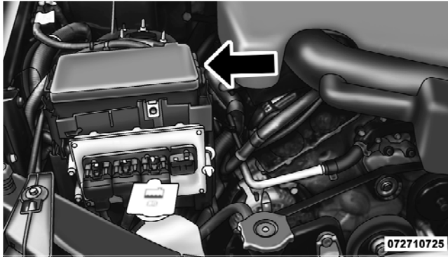
Totally Integrated Power Module
